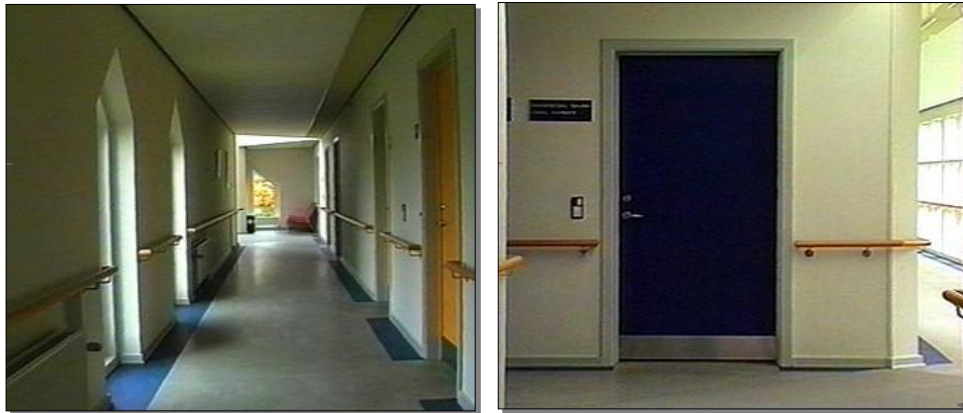
(Figure 2.2 illustrates a view to corridor side rails)
